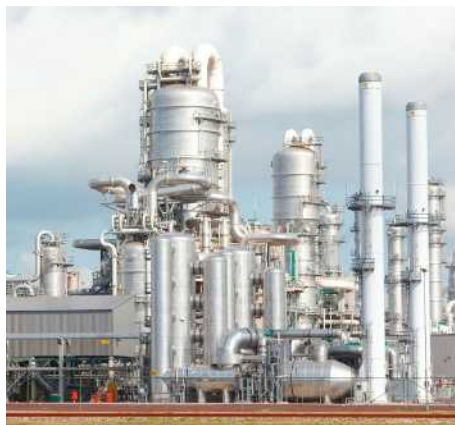
System expansion and post installation
